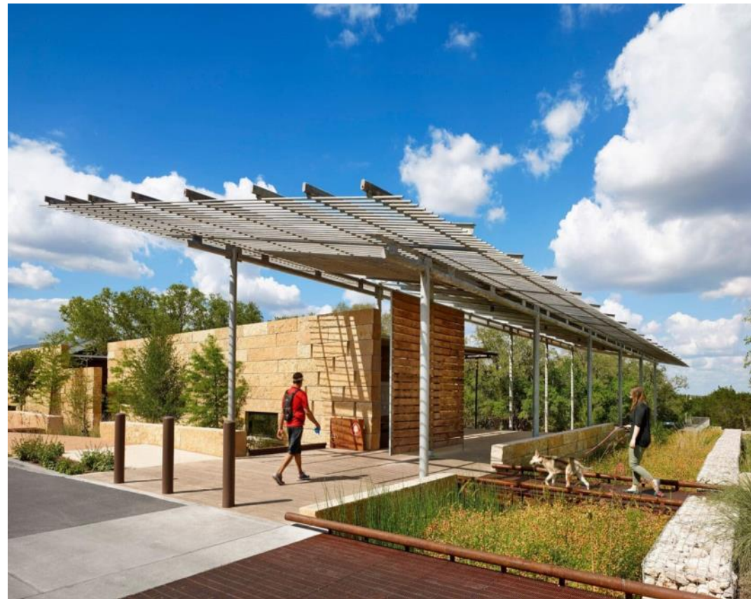
Exterior pavilion (with facilities)
